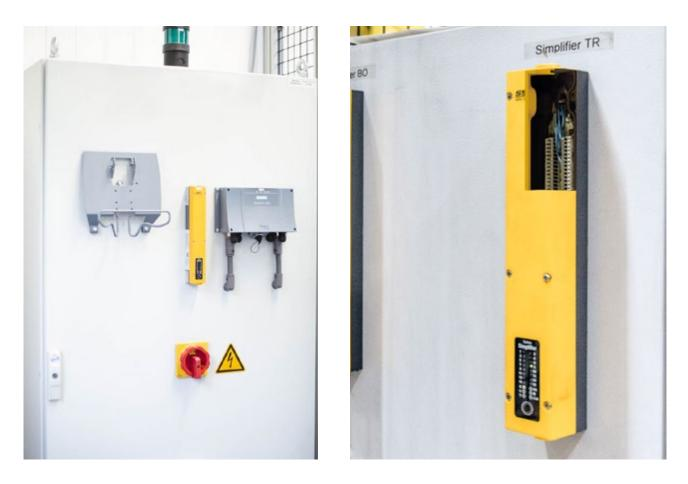
The Safety Simplifier is built onto a control cabinet from the outside, regardless of whether it is a cabinet for plant safety technology or a robot control cabinet.
